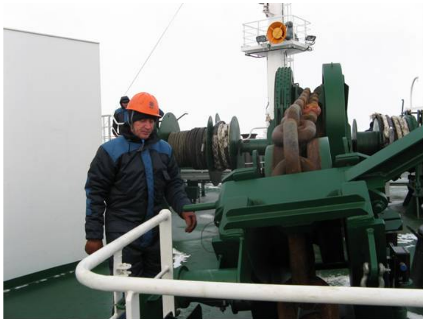
Figure 3-2 Anchor Windlass test
